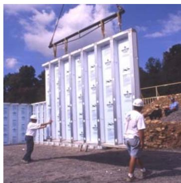
*Superior Walls* is America's leader in precast concrete foundation systems, with over 60,000 custom foundations installed nationwide.
